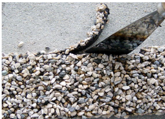
3 Cut off the fine gravel layer
