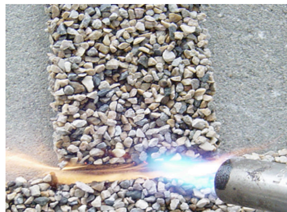
5 Short heating up of both ends
