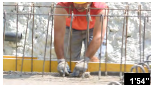
Incorporating BFL-Mastix waterstops type 20/40 R4 in fresh concrete of a raft
