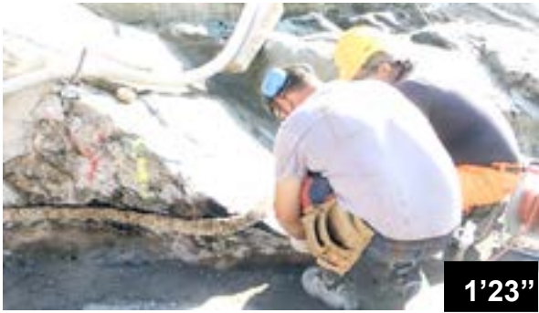
Gluing of BFL-Mastix bands on rock
