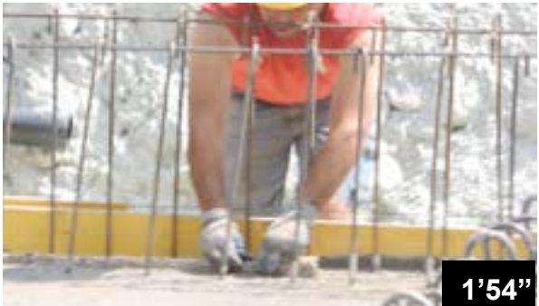
Incorporating BFL-Mastix waterstops type 20/40 R4 in fresh concrete of a raft
