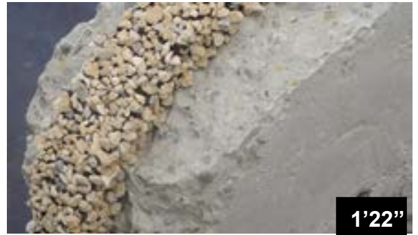
Gluing of BFL-Mastix bands on an irregular surface
