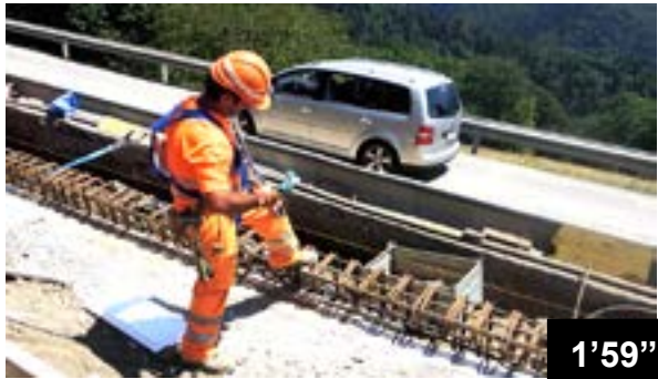
Height increasing a wall of a mountain road
