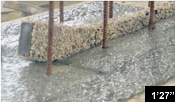
Placing of bands BFL-Mastix type R4 into fresh concrete
