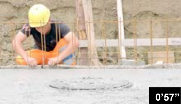
Incorporating BFL-Mastix waterstops in fresh concrete of a raft
