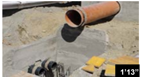
Gluing of BFL-Mastix bands on PVC pipes
