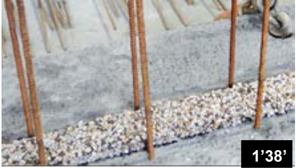
Horizontal gluing of bands BFL-Mastix type R
