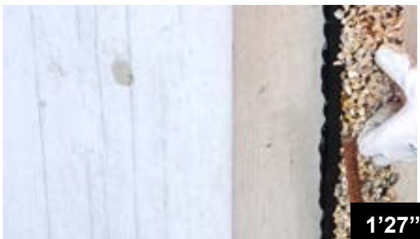
Vertical gluing of BFL-Mastix bands type R4 1/2 D
