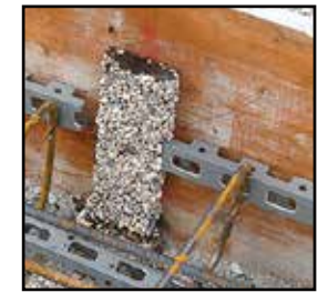
B2 Connection of bands black on black between horizontal and vertical bands
