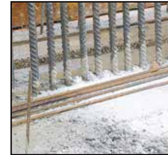
Introducing the BFL-Mastix bands type R4 into the fresh concrete
