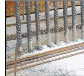
BFL-Mastix bands type R4 placed into the raft concrete
