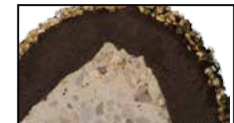
Adherence on hard concrete
